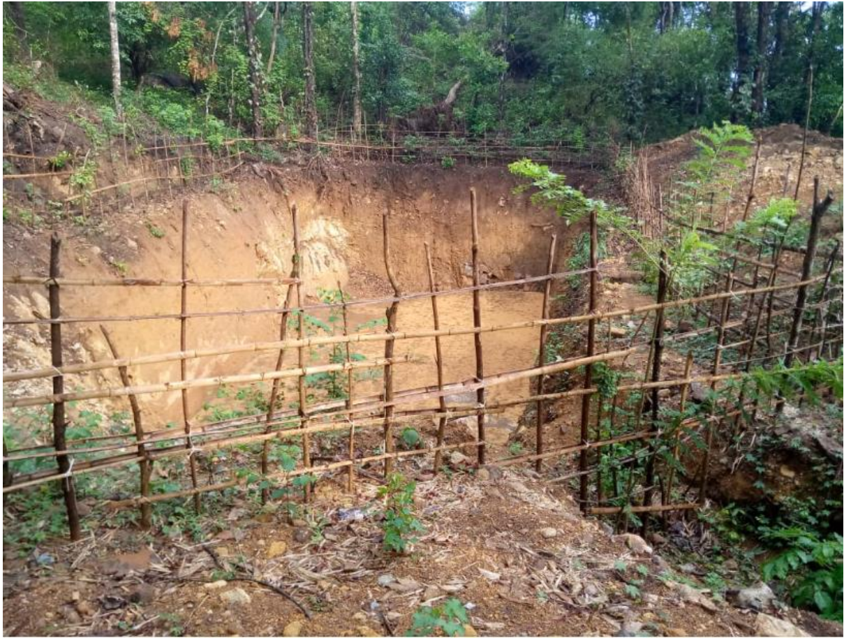
Plate G-1: Rain water harvesting Pond
